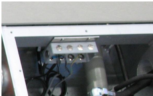
Image 18 - connection box inside cylinder housing
