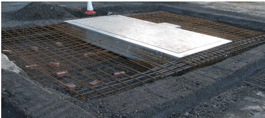
Image 6 – Wedge installation with reinforcement ready to pour the concrete
